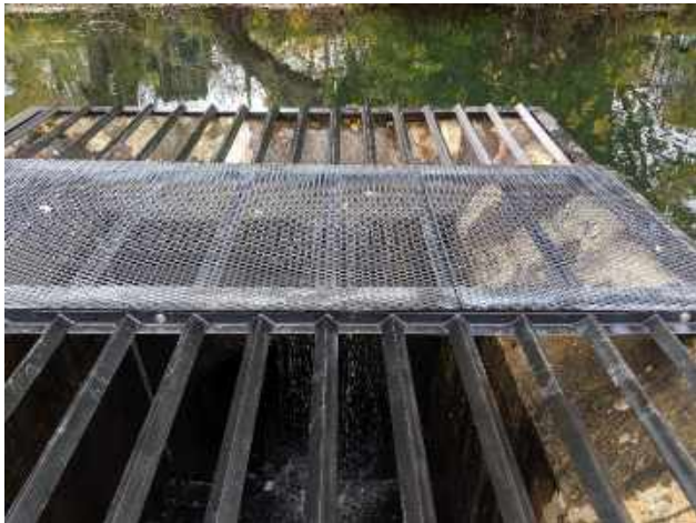
Principal spillway – new trash rack
