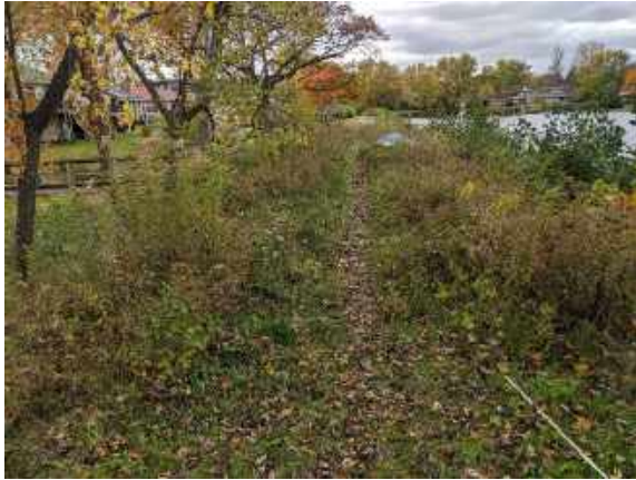
Poor dam vegetation coverage
