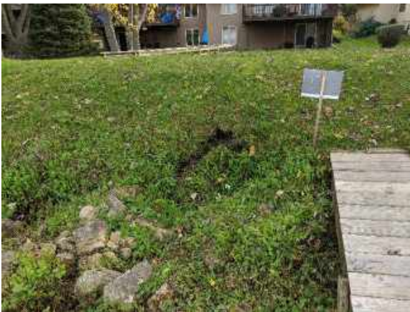
Sloughing on dam face, multiple locations. Mostly good turf coverage.
