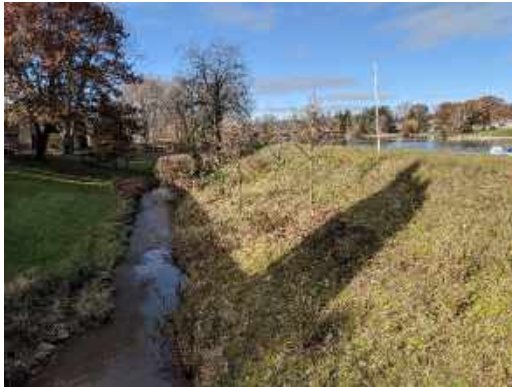
Newly planted oak trees, remove the three trees on the dam.
