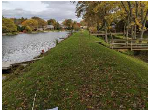
Sloughing on dam face, multiple locations. Mostly good turf coverage.
