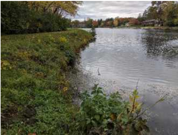
East end of dam, shoreline sloughing
