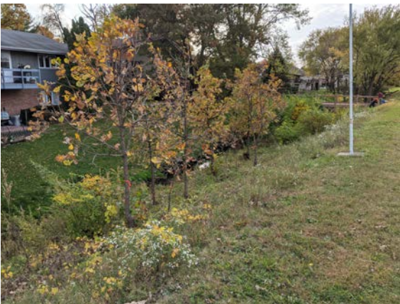
Tree removal on dam embankment.
