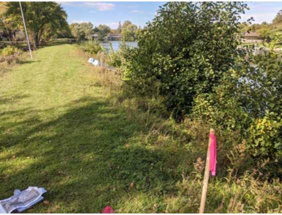
Woody plant material along bank must be removed.
