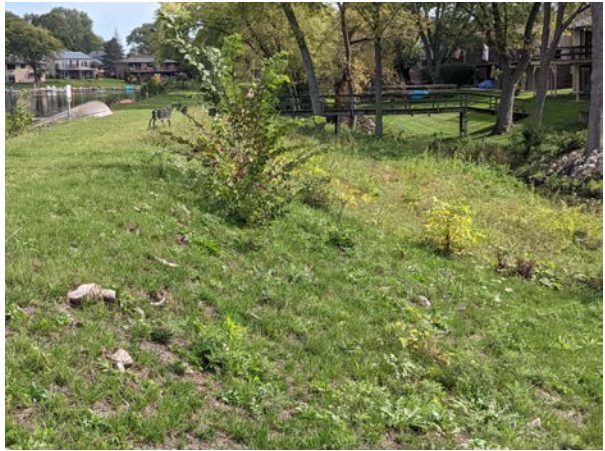
Some progress has been made on developing a turf surface for the dam. Woody plant material must be removed, stumps ground and backfilled with compacted soil.
