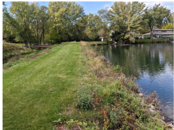
There is too much non-turf vegetation on the fore slope and backslope of the dam.
